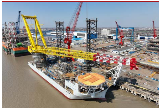
HEIGHT ADVANTAGE: The Voltaire under construction at Cosco in China is equipped with the world's tallest Huisman leg-encircling crane
