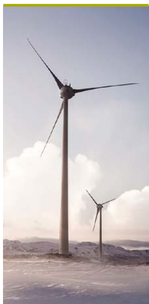
SYNERGIES: Test Enercon turbines installed near the Burfell hydropower plant
