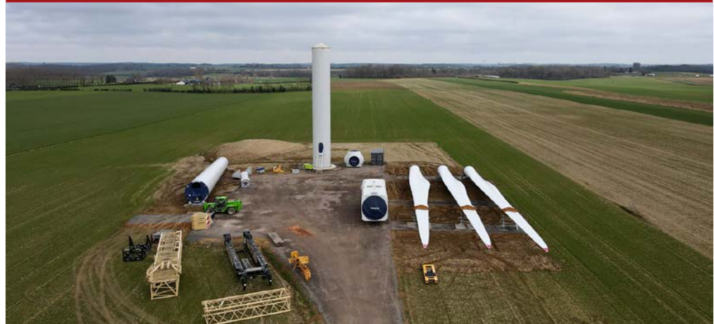
FRENCH FINISHING LINE: Falck Renewables has completed construction of the 12MW Illois wind farm in northern France's Seine-Maritime department. The last of six Vestas V90-2MW turbines with 80-metre towers went up in mid-April with the testing and commissioning phase now underway. Commercial operations are expected in July.
